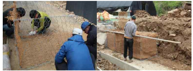
Assemble of revetment of using gabion systems with vegetation base materials
