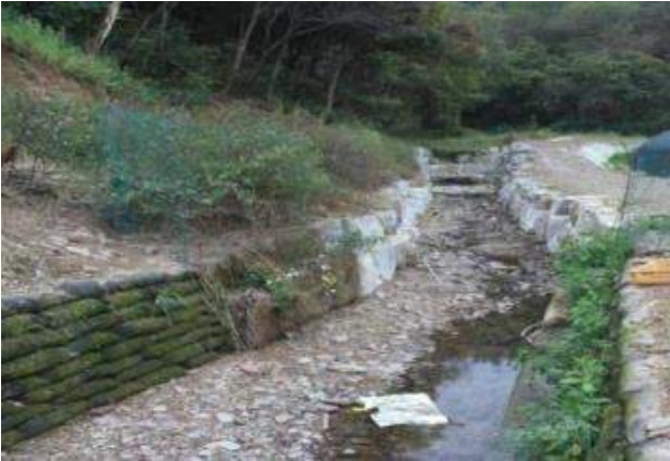
Fig. 3. Coverage of sack of revetment, revetment of using gabion systems with vegetation base materials and stone revetment
