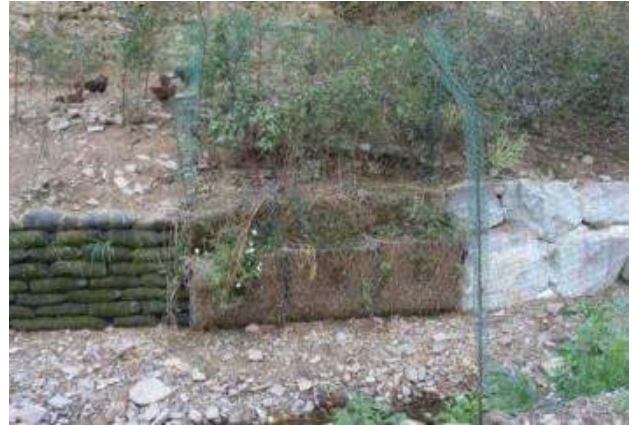
Fig. 3. Coverage of sack of revetment, revetment of using gabion systems with vegetation base materials and stone revetment
